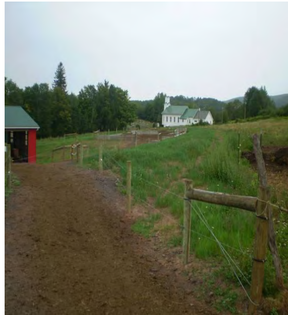
Photo Taken After Construction
