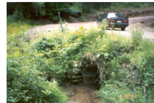
Stream Crossing Problems Corrected by Installation of New, Larger Pipe
