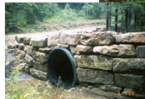
Stream Crossing Problems Corrected by Installation of New, Larger Pipe
