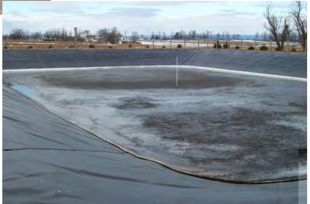
HDPE lined Storages
