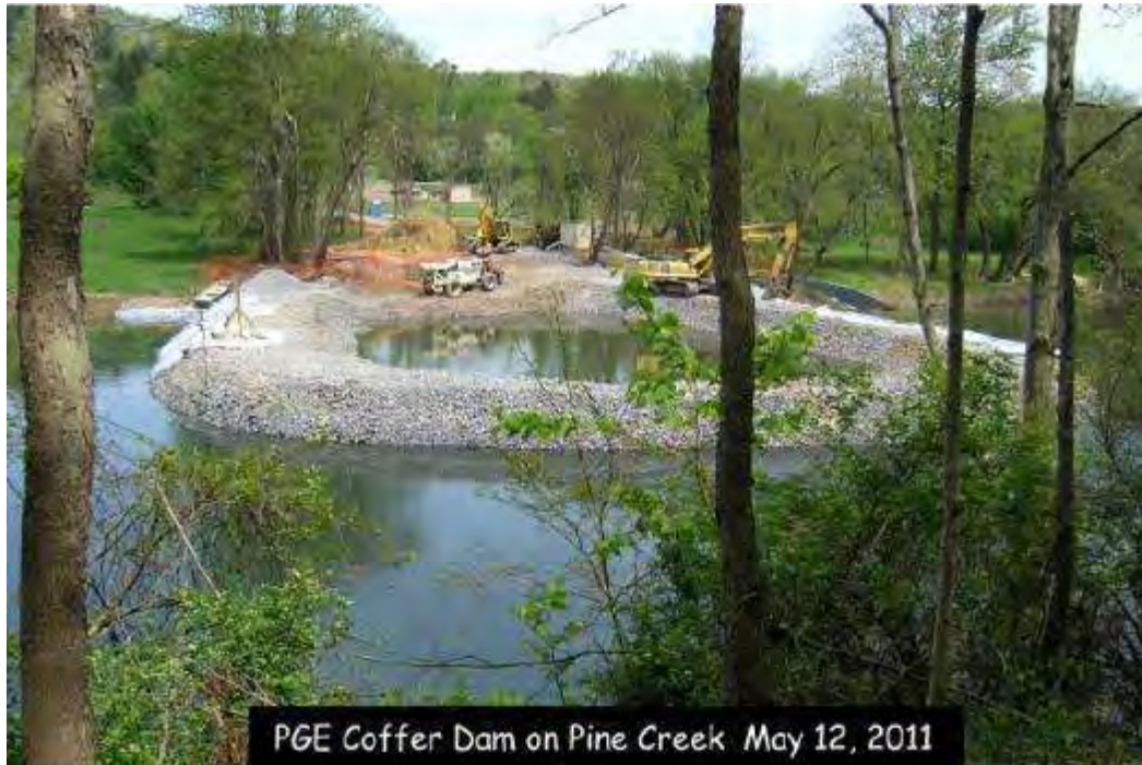
PGE Cofferd Dam on Pine Creek May 19, 2011
