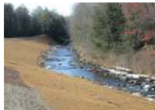
Stream Channel (After)
