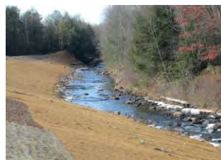
Stream Channel (After)
