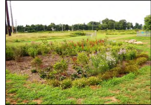
Perkiomen Stormwater Improvement Project
