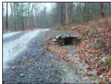
Above: Shallow Cross Pipe
