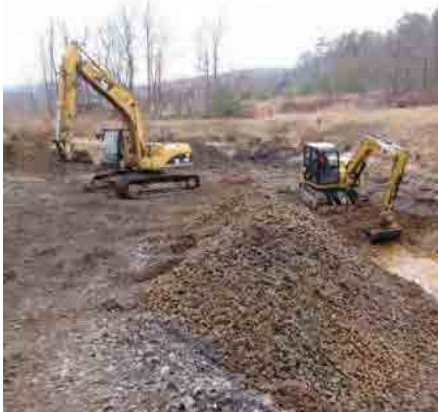
Rehab and reconstruction of Oven Run AMD Passive Treatment Site E and Site F on the Stonycreek River
