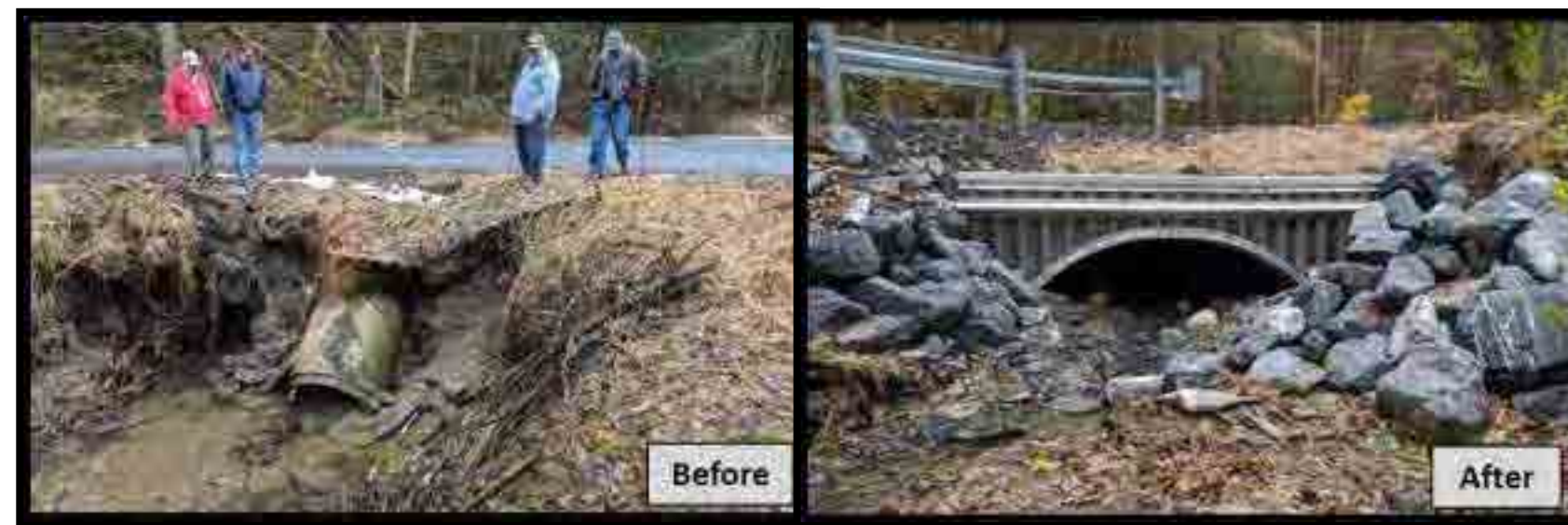
Ponderosa Road Stream Crossing Replacement – this Dirt and Gravel Road project reduced sediment in Stone Creek and improved safety on this township road
