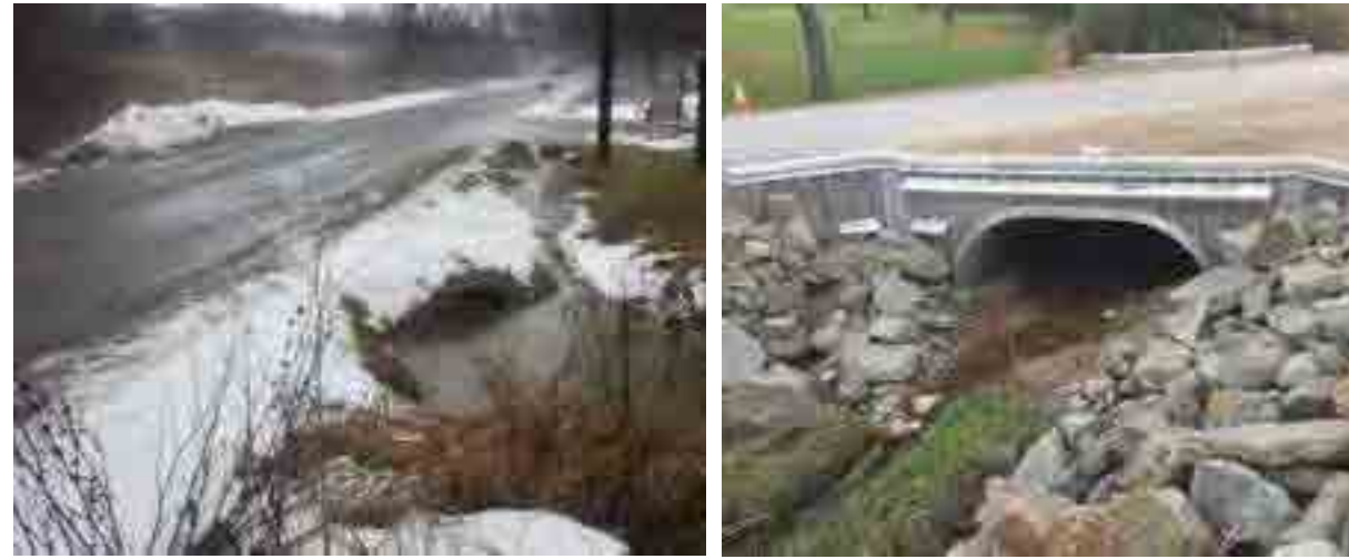
Outlet before (above left) and Inlet after (above right)
