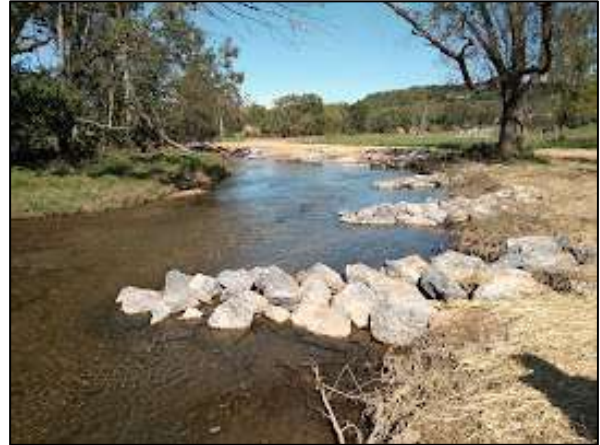
[After] A series of rock "barb" deflectors on the Cacoosing Creek.
