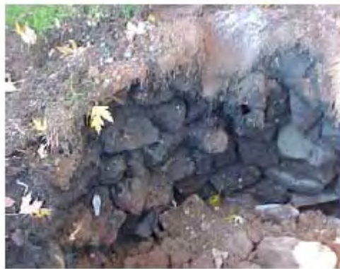
Figure 4. Collapsed Cesspool
